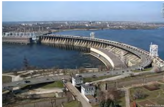
Fig. 2. Drainage dam of the Dnipro HPP.
