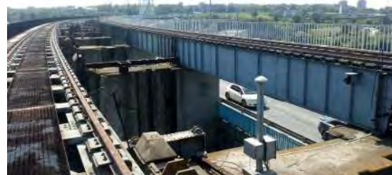
b – monitoring point MP-4
