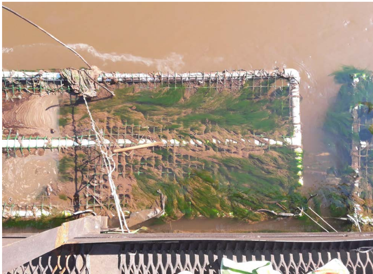
Fig. 1. Rafts with fibrous carrier of the “VIYA” type installed at the sludge collector of the “Zaporizhstal” PJSC plant
